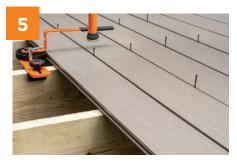
**FASTEN EVERY JOIST** Fasten all of the remaining clips at each joist.
