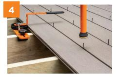
LIFT UP TOOL After fastening, lift up on the tool to return your drill to starting position.
